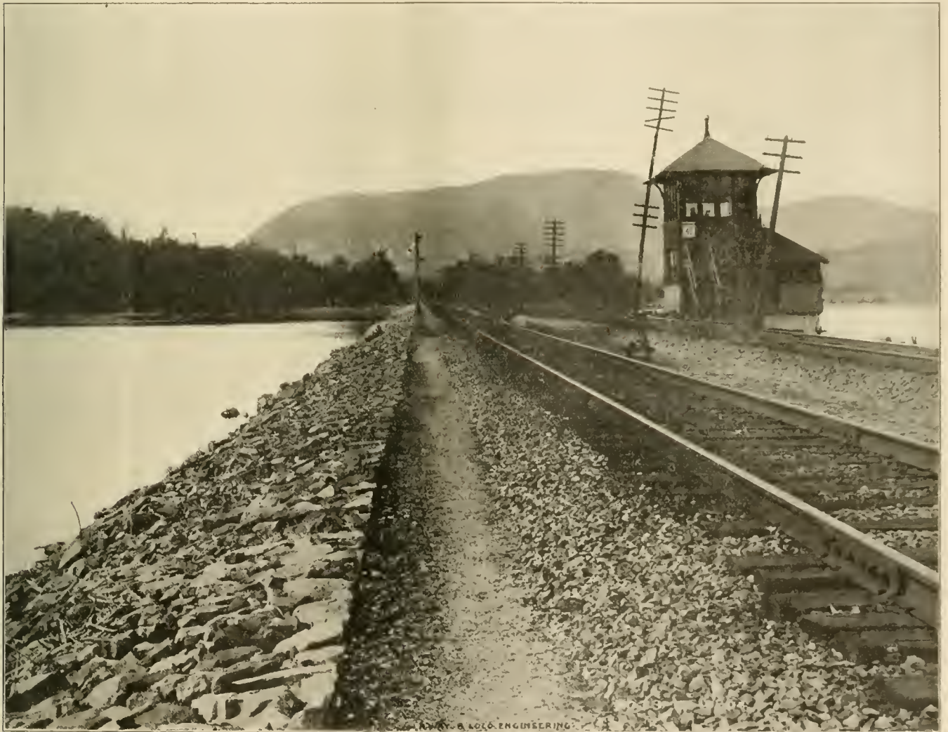
TYPICAL BLOCK SIGNAL TOWER ON THE NEW YORK CENTRAL & HUDSON RIVER RAILROAD.
